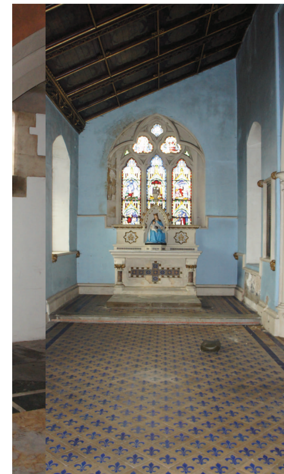
THE LADY CHAPEL TILED FLOOR EXPOSED
