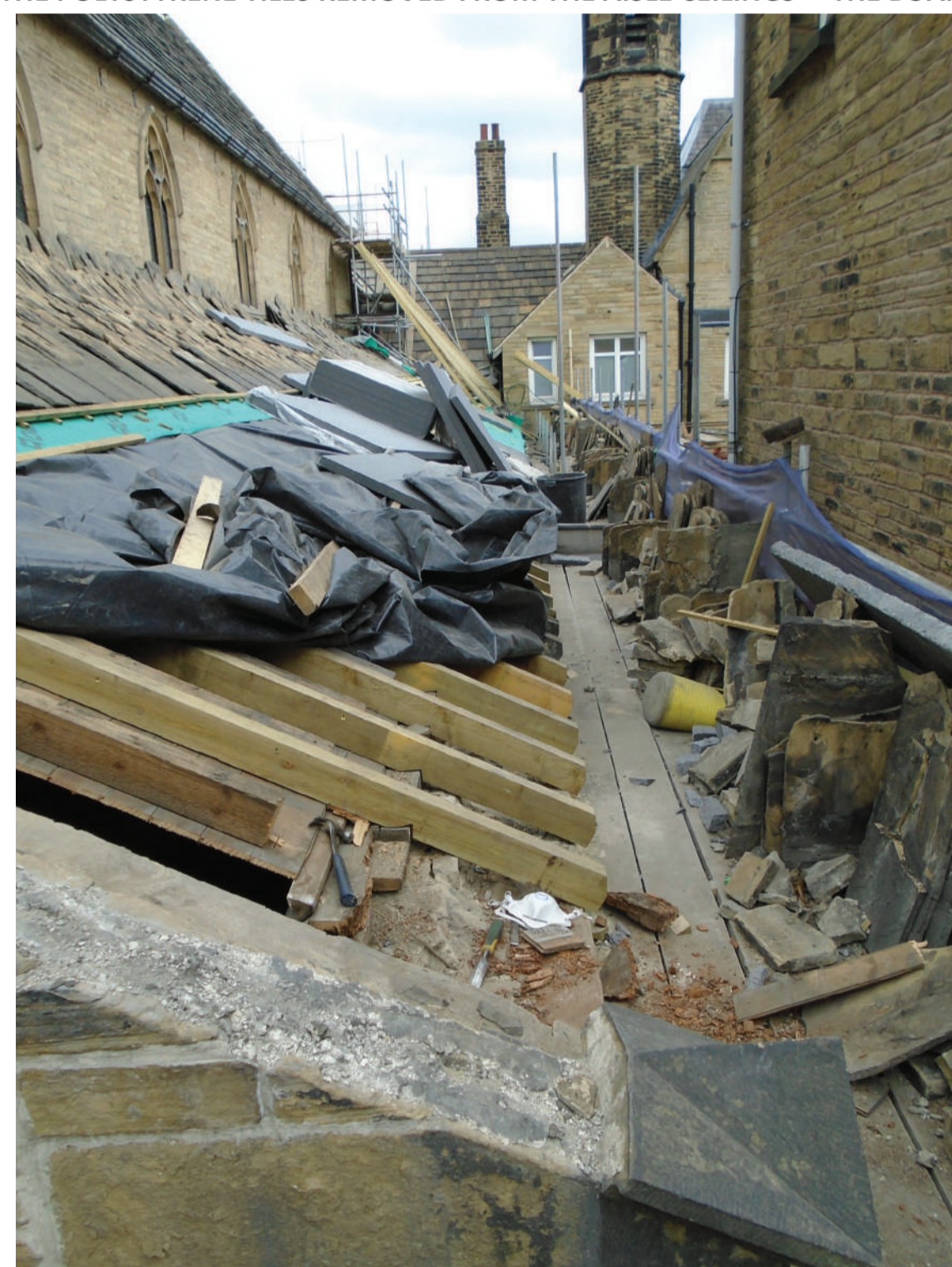
THE AISLE ROOFS REPAIRED, INSULATED AND RE-SLATED
