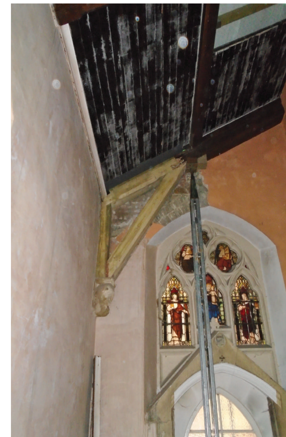
REPAIRS TO THE RAFTERS UNDERTAKEN
