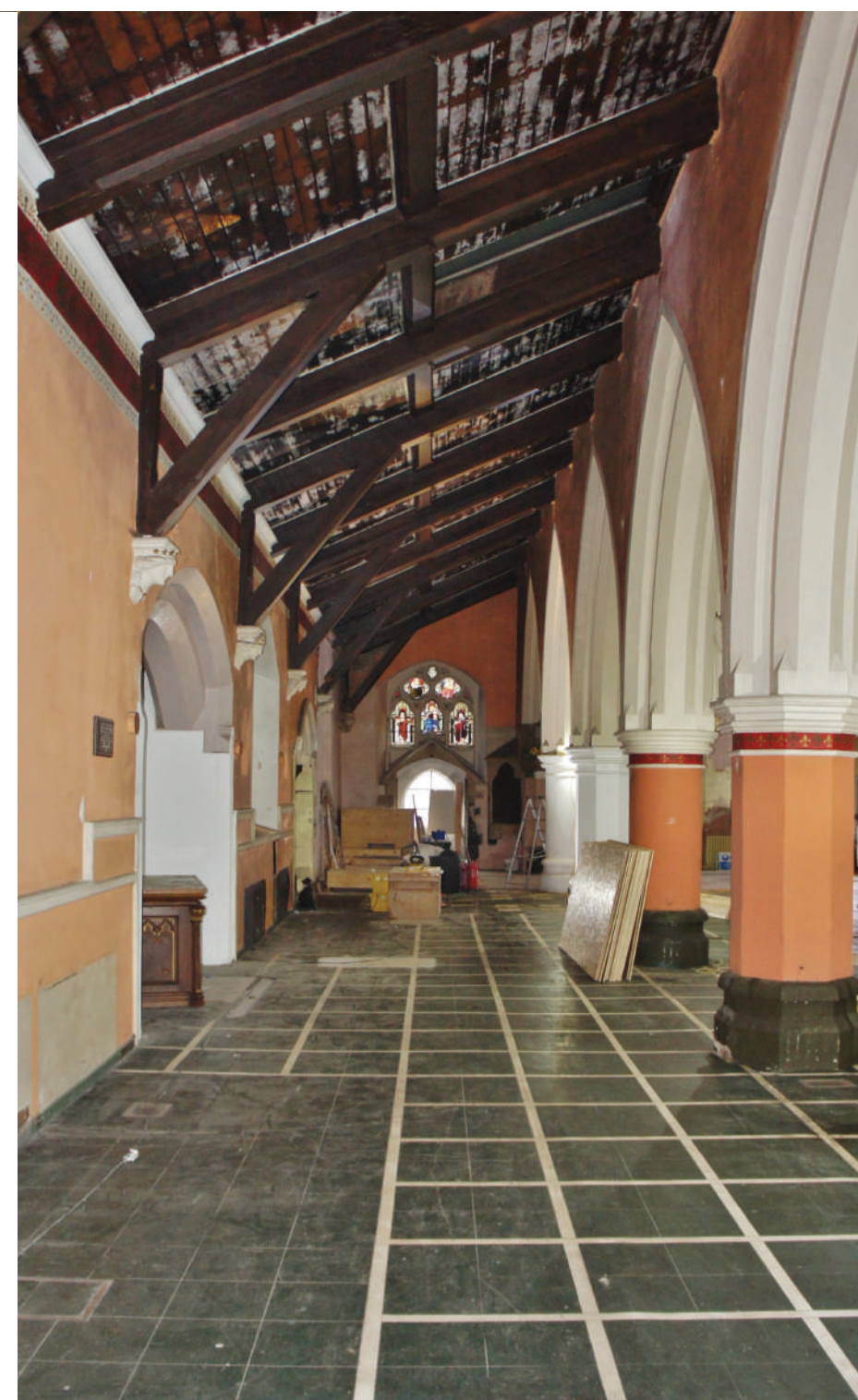
THE POLYSTYRENE TILES REMOVED FROM THE AISLE CEILINGS
