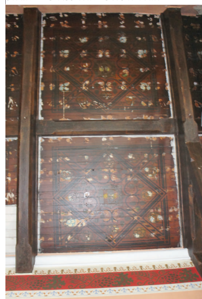
THE AISLE CEILING DECORATION EXPOSED
