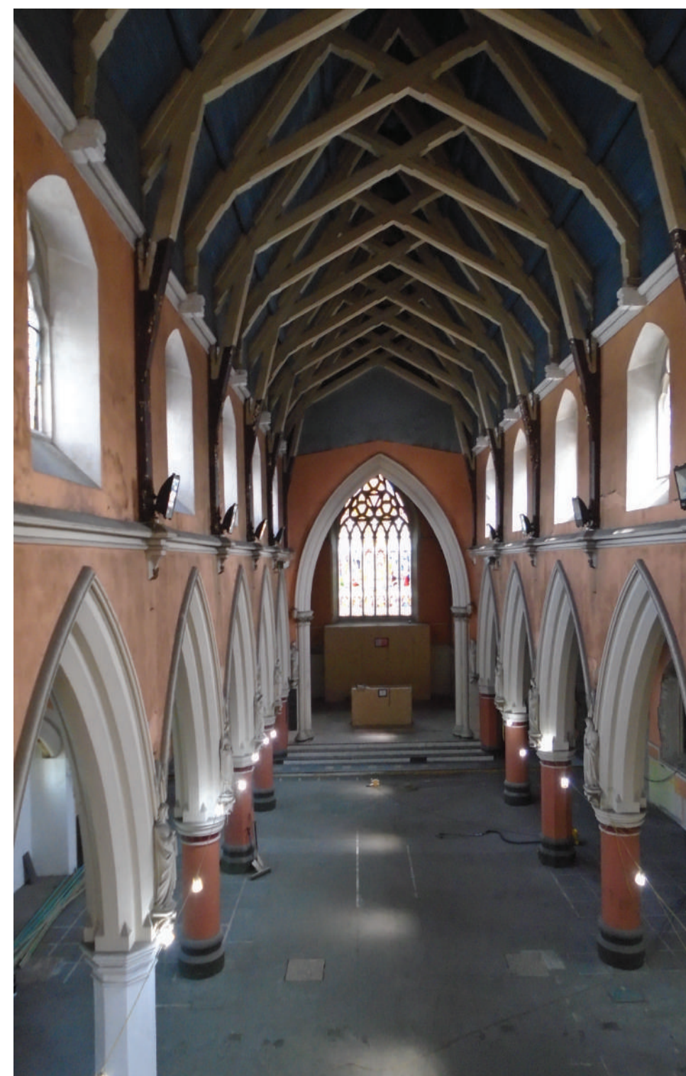
THE NAVE CLEARED AND THE SUSPENDED CEILING REMOVED
