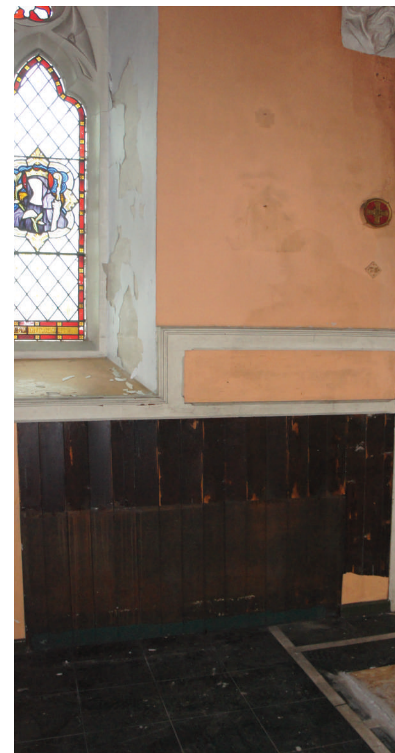
THE BOARDING EXPOSED IN THE AISLES
