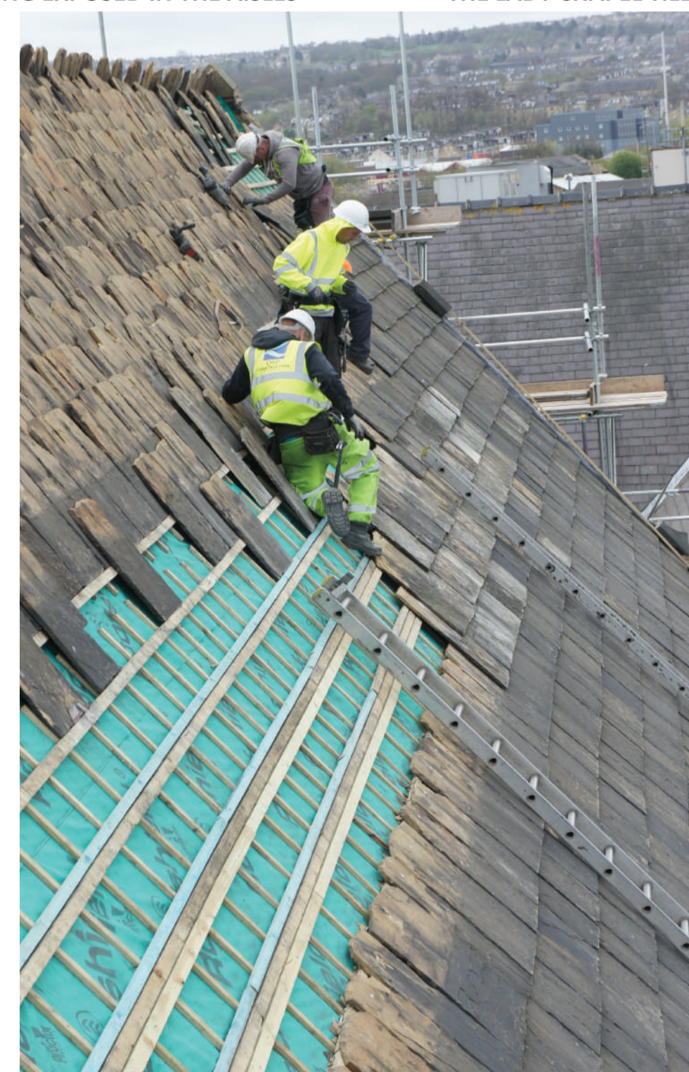
THE NAVE ROOF RE-SLATED AND INSULATED
