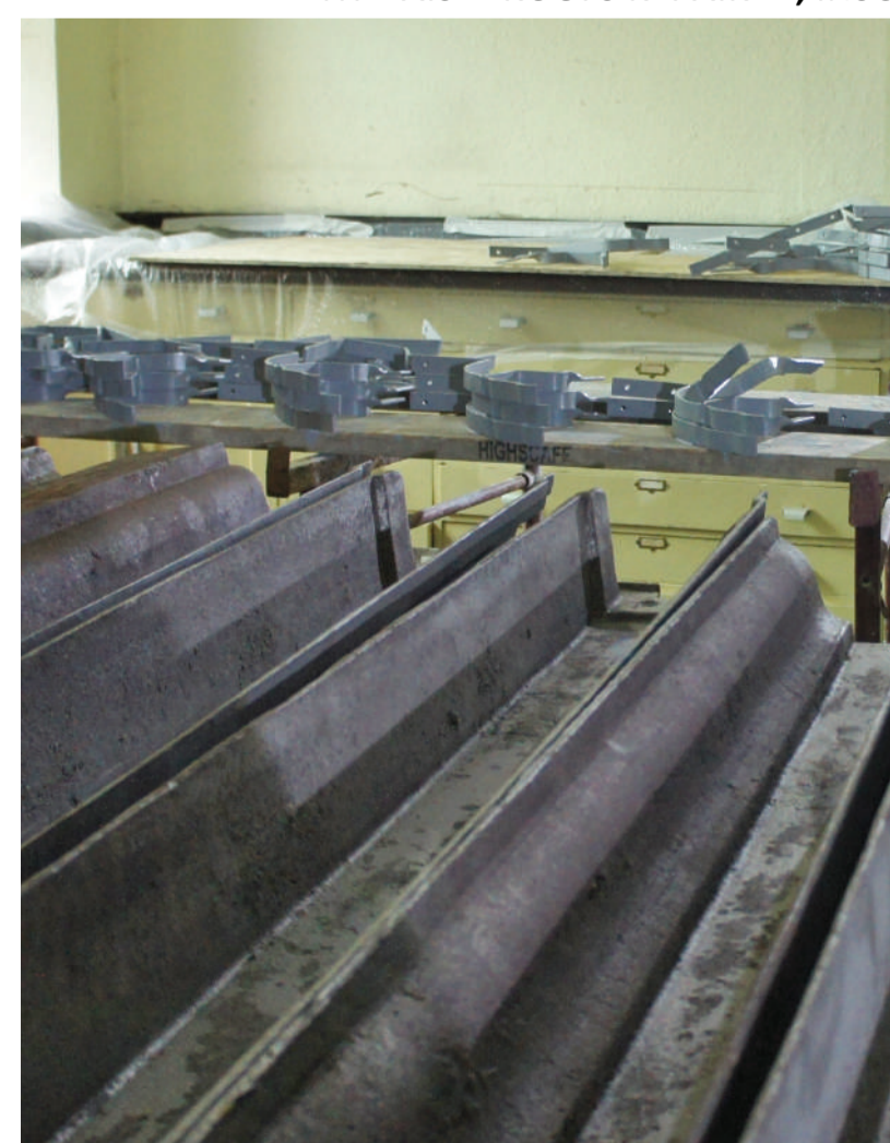
THE IRON GUTTERS REPAIRED AND RE-DECORATED
